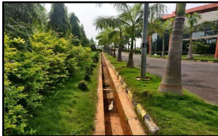
Storm water drains at IKSEZ Office building
